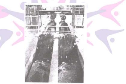
ii) Wat er then goes to a grit and sand removal tank. The speed of waste wat er is decreased to allow sand, grit and pebbles to set the down.
