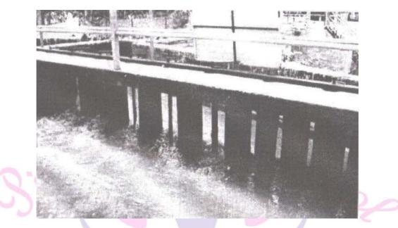
iii) The water is then allowed to settle in a large tank sloped towards the middle. Solids like faeces settle at the bottom and are removed with a scraper.
